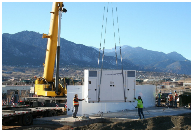
Battery storage being installed at Fort Carson, Colorado. Credit: Scott Clark via U.S. Army Corps of Engineers, CC BY-1.0
