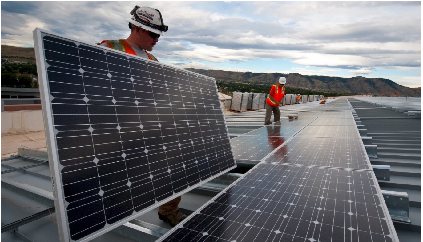
Solar panels being installed on a rooftop. Credit: skeeze via pixabay, CC-BY-1.0
